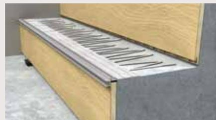
3. Apply glue to the sub-profile and the step. Spread out the glue across the sub-profile.
