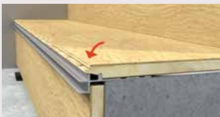
4. Place a plank on the step against the rising edge of the sub-profile.
