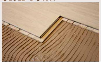
Quick-Step Timber can also be directly adhered to a well prepared sub floor. Whilst direct sticking wood flooring has some advantages (reduction of foot sound), there are also disadvantages that need to be considered. More information can be obtained at your local Quick-Step dealer.
