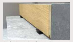
Glue the plank to the riser. The spacers ensure that sufficient space is left underneath to fit in the step.
